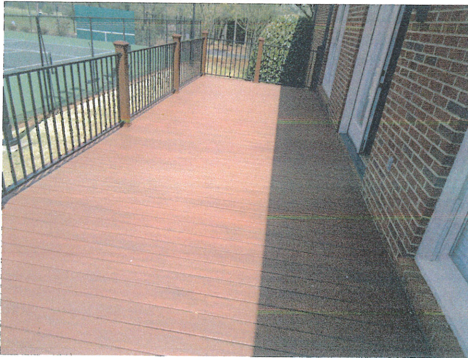
Photo #4 New deck
