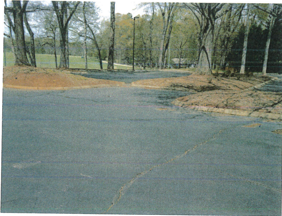
Photo # 11 Parking Area Conditions
